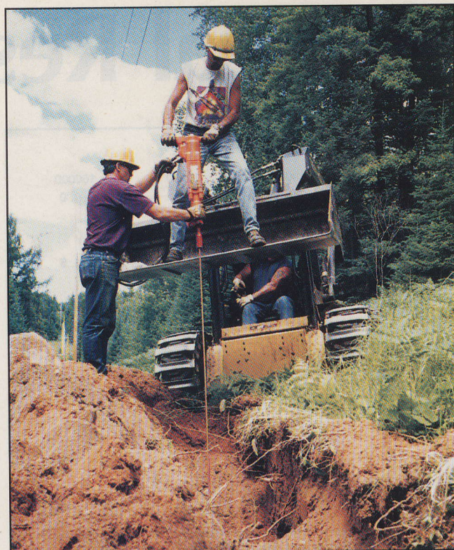
Fig. 5. Hammer on top of driven rod being handled by a worker standing on a raised plow.
