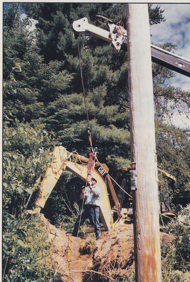
Fig. 4. Hammer on top of driven rod and suspended from a crane.
